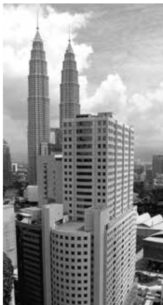
UOA Centre I & II, Kuala Lumpur
