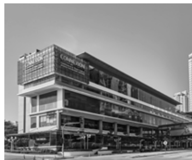
Connexion Conference & Event Centre, Bangsar South
