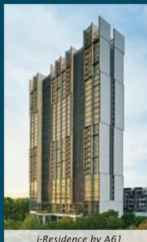
i-Residence by A61
