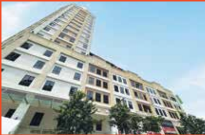
Hotel Sentral Kuala Lumpur @ Brickfields Hotel Development
